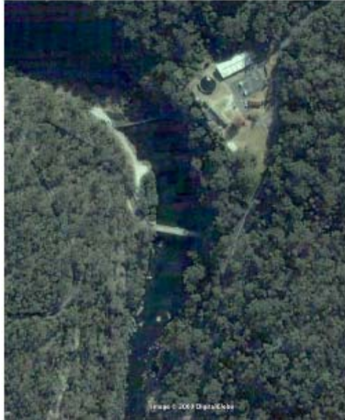
Broughtons Pass Weir, Google Earth image
