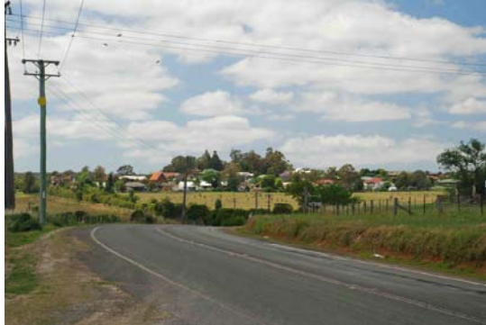
Menangle Conservation Area viewed from the west.
